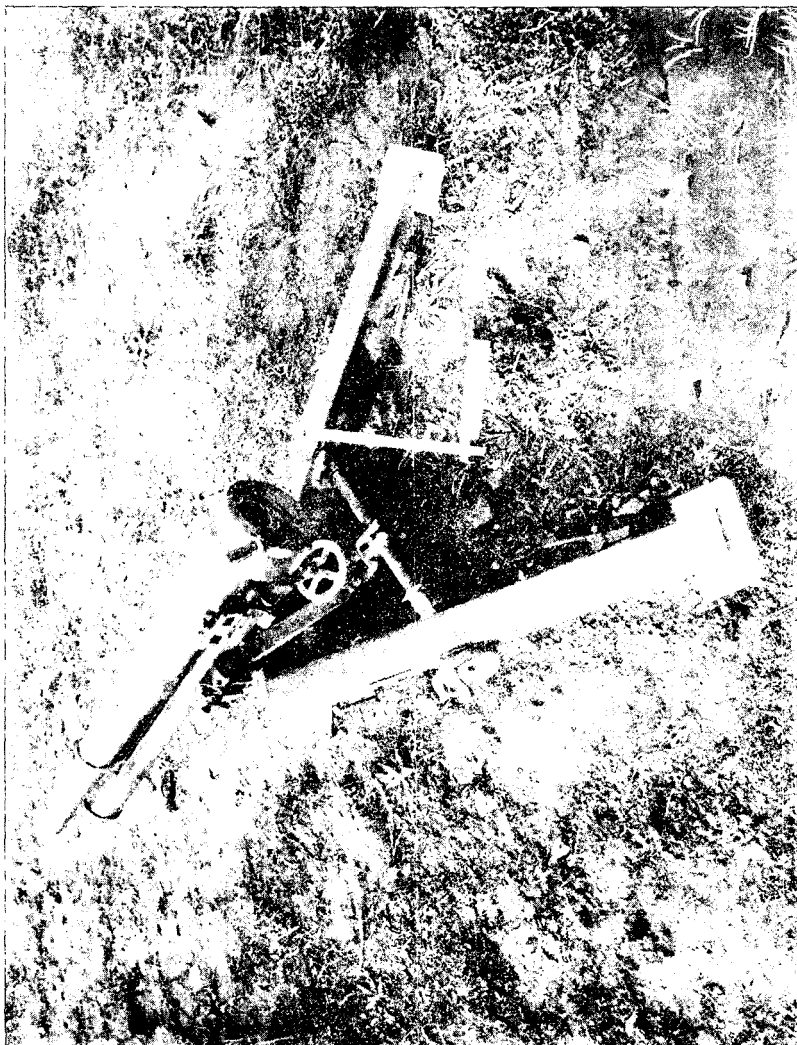
FIGURE 4. - GUN, 37-MM, M1916, ON CARRIAGE, M1916A2.
